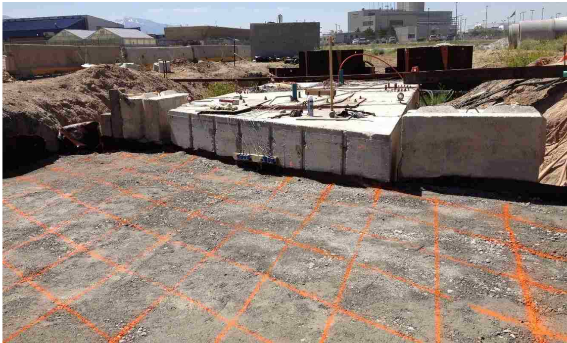
Figure 3-16. Grid painted at 2 ft by 2 ft (0.61 m by 0.61 m) spacing prior to 30° skew GRS test.
