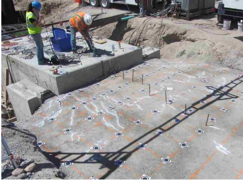
Figure 3-17. Backfill instrumentation and inclinometer readings following 0° skew gravel test.
